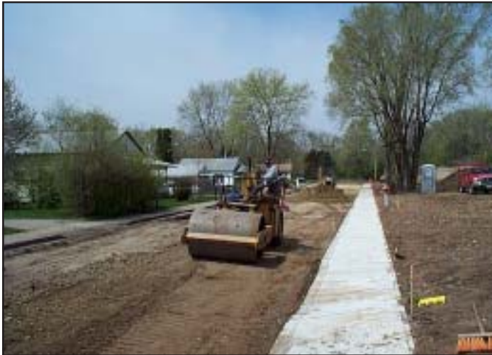
Reconstruction usually results in significant disruptions
